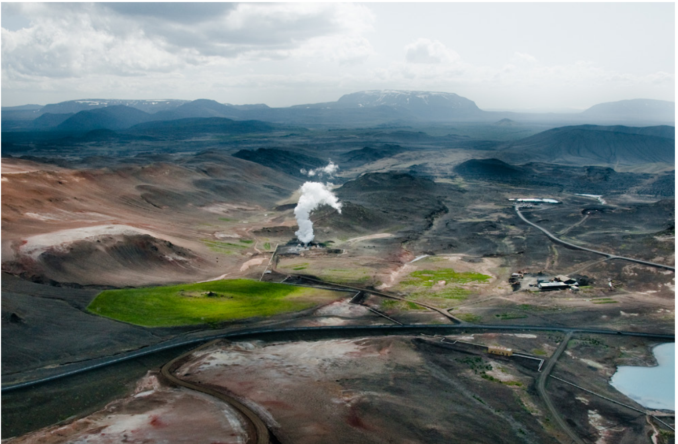
Bjarnarflag power station
