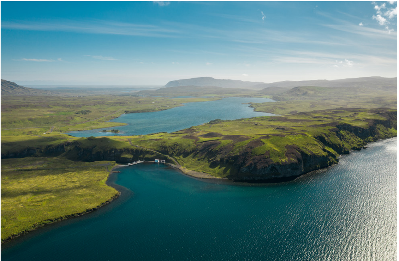
The dam and intake of Steingrímsstöð power station
